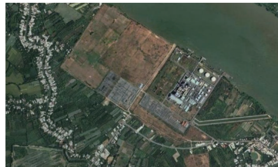
Satellite view of the O Mon Power Complex along the Hau River in Can Tho City, Mekong Delta Region. The 3.81-GW O Mon Power Complex will be fueled by the gas extracted from the JBIC-funded Block B gas field project off the coast of Kien Giang province in Vietnam. (Photo taken from Google Maps, ©2024 Airbus, CNES / Airbus, Maxar Technologies)
