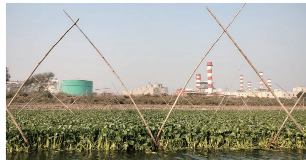
Meghnaghat Gas-fired Power Plant ©CLEAN, Bangladesh
